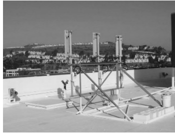
Antenna on roof, concealed behind a parapet
